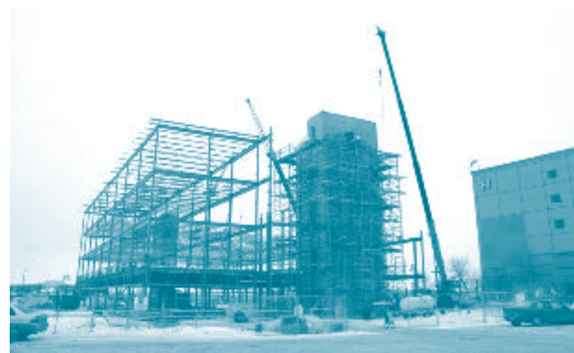
Construction of the Day Support Building at the Grey Nuns
